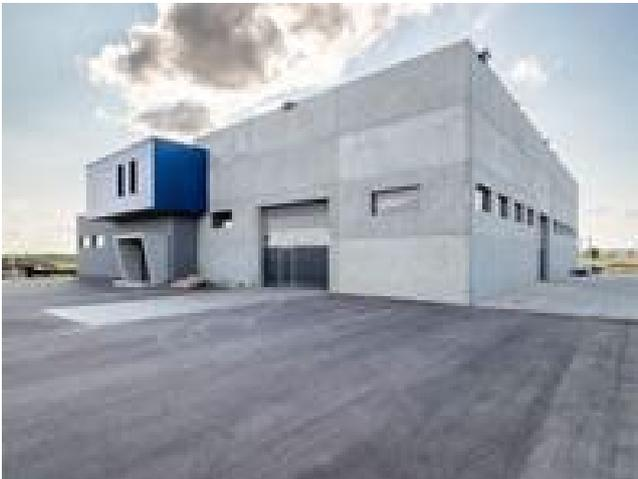
*The high-quality concrete facade featuring the natural stone look of the new precast plant was made possible thanks to the use of Schöck Isolink.*
