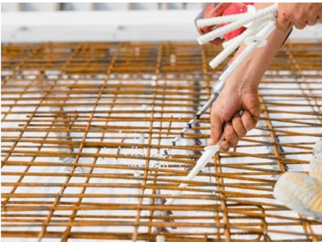
*The Schöck Isolink Type C-SD for freely suspended outer shell panels is set into the insulation at a 45-degree angle.
