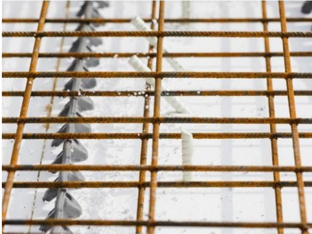
*The plastic depth limiter is installed on the Schöck Isolink to secure the insertion depth.*
