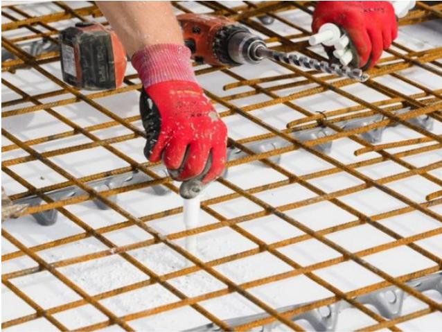
*The Schöck Isolink Type C-SH for the attached outer shell panel is set into the insulation at a depth of at least 6 cm.
