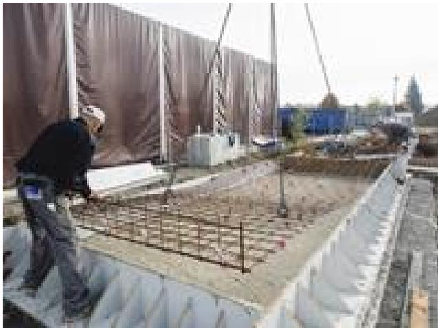
*Installing the reinforcement elements on the outer shell panel.*
