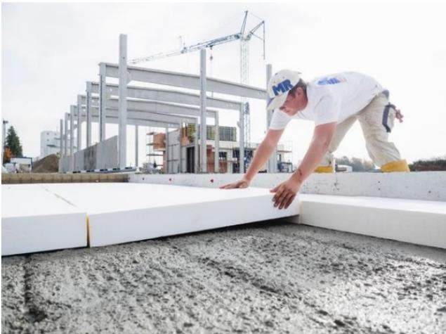
*The insulation layer made of expanded polystyrene (ESP) comes after the
