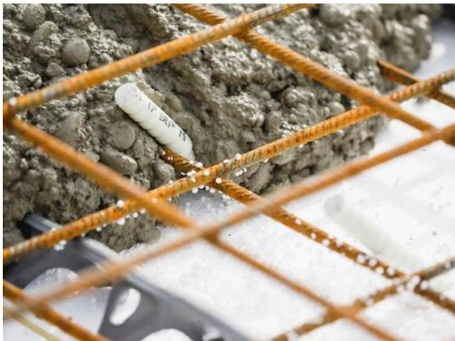
*The load-bearing shell panel is concreted as the last layer.*
