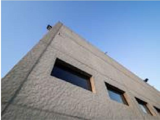
*Façade elements with a load-bearing shell panel made of concrete (15 cm), insulation made of expanded polystyrene (12 cm), and an outer shell panel (8 cm).*
