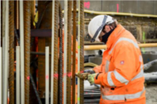
*The overlapping joints between the individual cages were secured using wire rope grips.*
