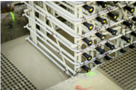
*Combar was used as the reinforcement material instead of steel. It is a glass-fiber-reinforced polymer (GRP) specially developed and produced by Schöck, which, unlike steel, can be easily machined.*
