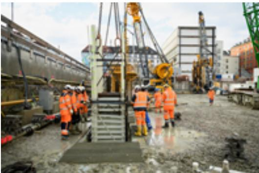
*In the soft-eye area, reinforcement cages made of Combar were placed throughout a 24-meter area.
