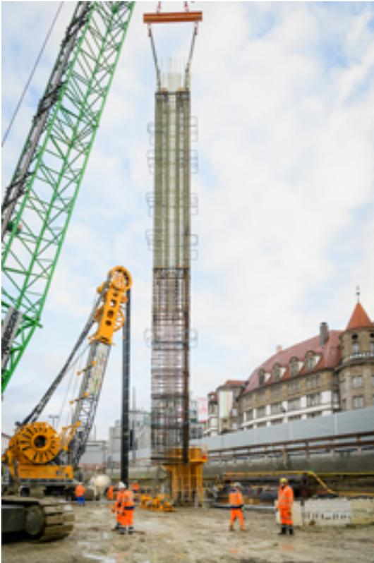
*The special 18-meter length of the Combar bars proved to be advantageous for the construction of the shaft walls, because this allowed for the construction of only one reinforcement cage.
