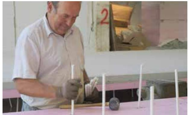
2. Insert the Thermoanker into holes drilled into the thermal insulation
